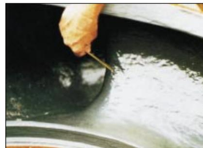
ARC Composites now resist the corrosive, abrasive slurry, lengthening the maintenance interval. Smoother surface improves flow.
